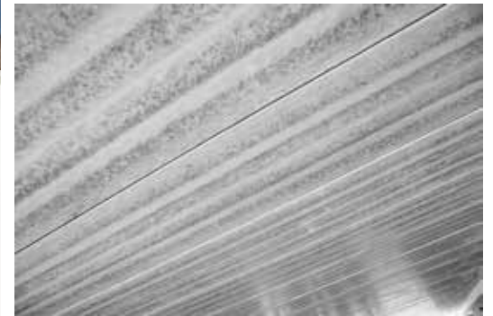
Hollowcore slabs can be used as finished ceilings
